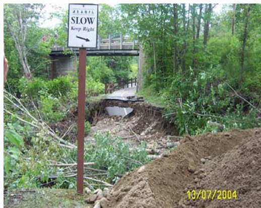
In July, 2004, significant rains caused devastating erosion along the Stowe Bike Path. The path has been re-routed several times to accommodate a river that needs access to its floodplain.
